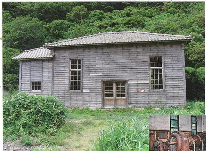
Tojigawa Hydro Power Plant No.2
