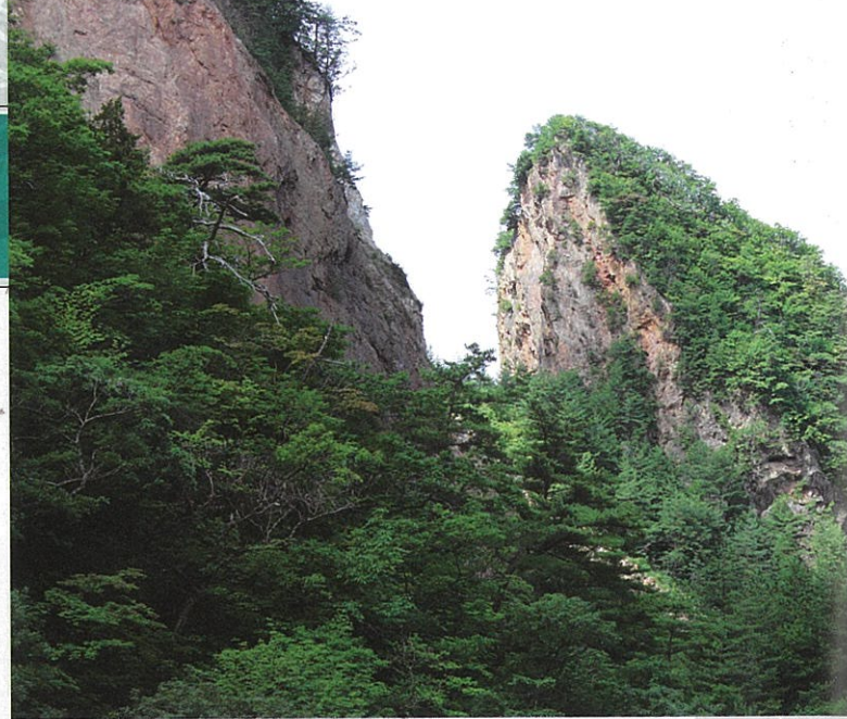
Doyu-no-warito Open-cut from the east
